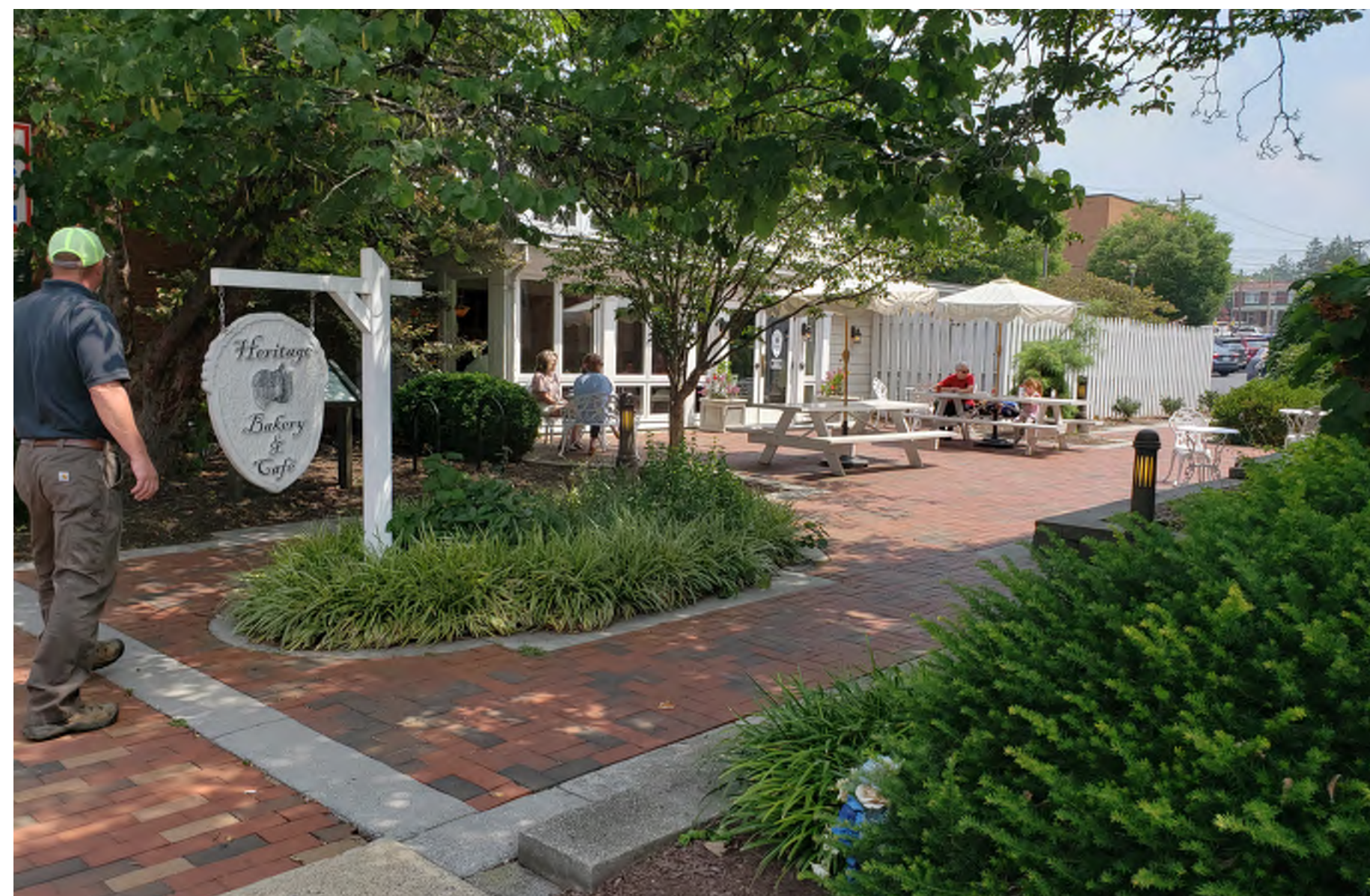
8. Primary entrance view of the Hardesty-Higgins House Visitor Center, marking a key arrival point of a special destination within the downtown district.
