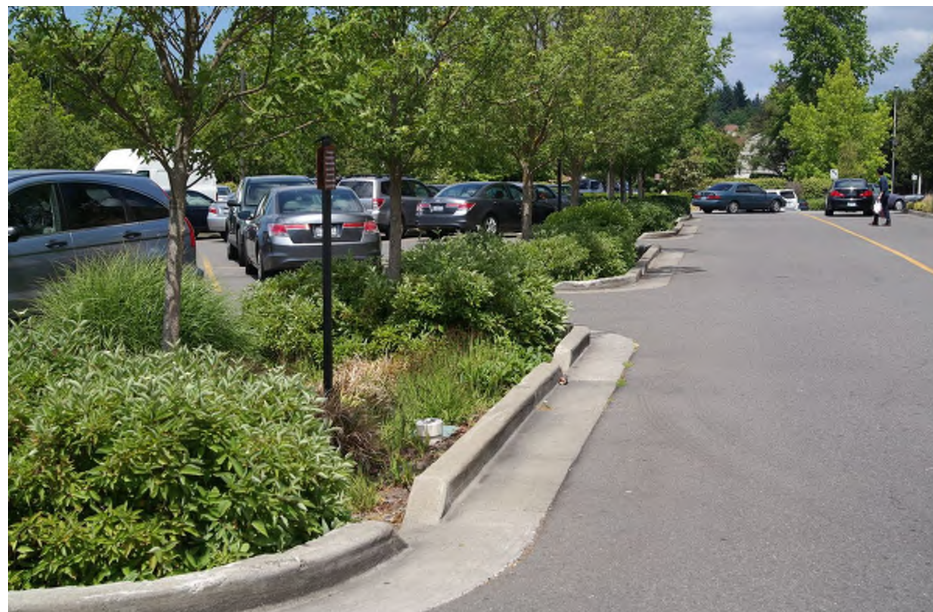
1. Terminal and interior islands help direct drivers, reduce driving speeds within parking lots and help reduce runoff.
