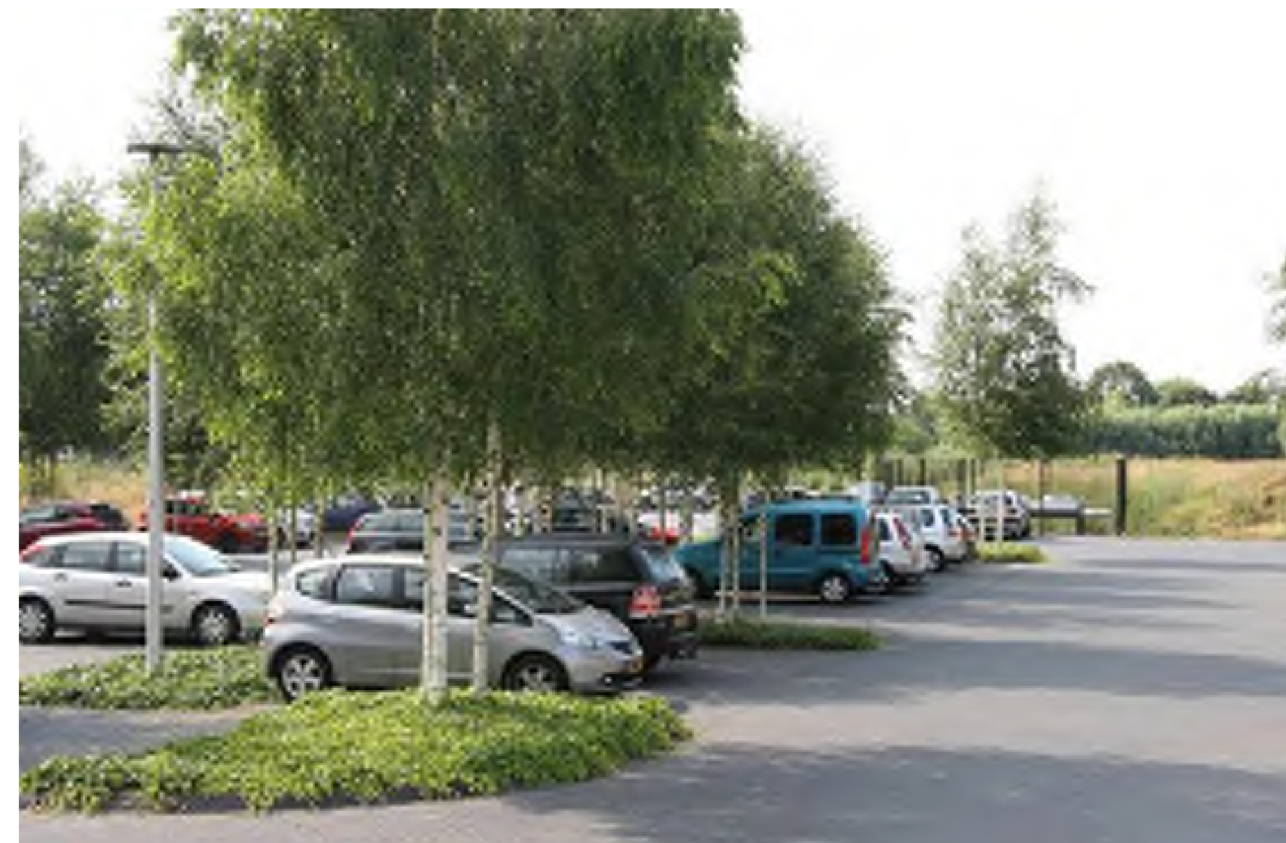
2. Terminal and interior islands help direct drivers, break up the expanse of asphalt in parking lots and reduce negative visual impacts of large parking lots.
