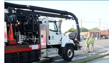
Storm Drain Cleaning
