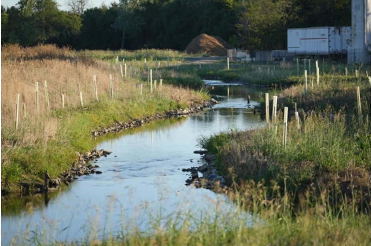
The Blacks Run stream restoration project in the southern part of the City restored just over a mile of stream, reducing streambank erosion and restoring habitat. It helped remove approximately 2,400 pounds per year (lb/yr) of TN, 1,100 lb/yr of TP, and 123 tons/yr of TSS from the Blacks Run watershed.
