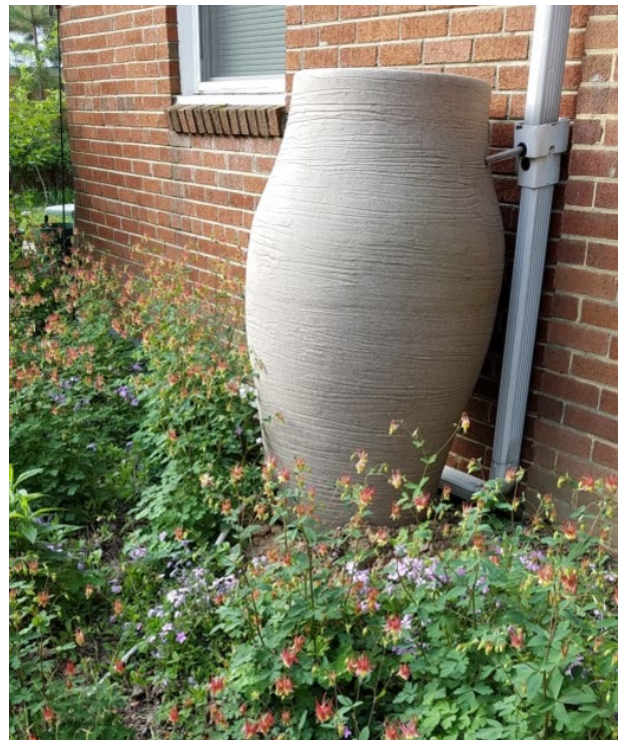
Rain barrels are a common residential BMP. They collect rain runoff from roofs, preventing the runoff from entering storm sewers. The collected water can be used to water plants.
